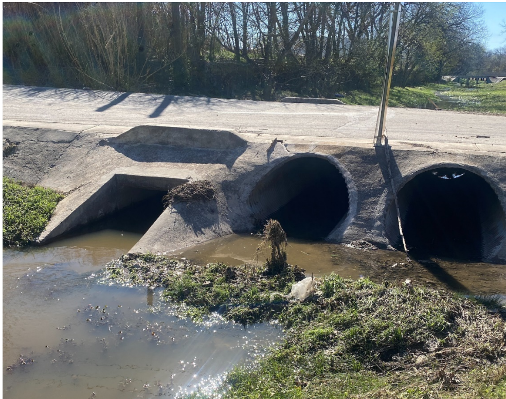
Figure 3 – Site Photo: McKie Street Crossing Downstream Face
